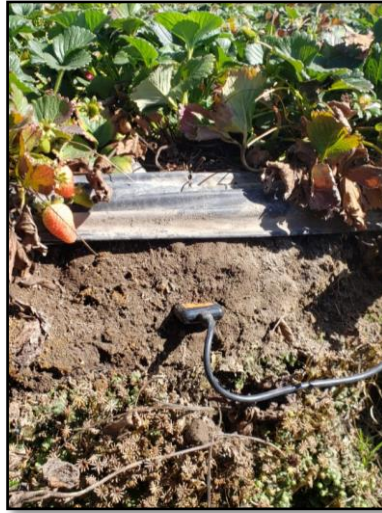
Fig. 11. Sensor installed on the ground horizontally.
