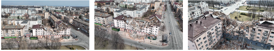
Fig. 2. Examples of drone imagery for Chernihiv Hotel “Ukraine”, damage level 3.
