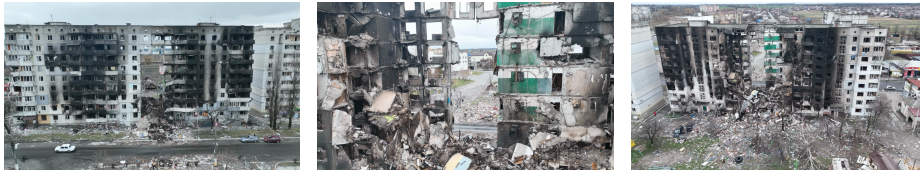
Fig. 1. Examples of drone imagery for Borodyanka, damage level 4.
