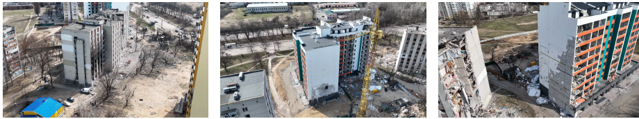
Fig. 3. Examples of drone imagery for Chernihiv residential area, damage level 2.
